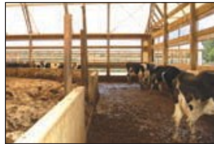
FEED SEPARATELY: A feed alley separated from the compost area by cement walls allows the compost to stay intact and the alley to be scraped.
